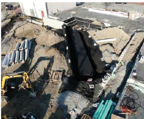
Underground Storm Water Detention System Example
